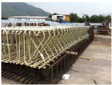
Bends in Pulwell GFRP Rebar are fabricated by shaping over a set of molds or mandrels prior to curing of the resin matrix. Field bends are not allowed. All bends must be made at the factory. All GFRP rebars exhibit a strength reduction through the bent portion of the rebar, which is recognized by all the consensus design guidelines. Research has shown that bends typically maintain 38% to 50% of ultimate tensile strength through the radius.
