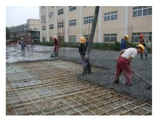
There are a number of authoritative consensus design guidelines for the designer to follow. Generally the design methodology for FRP reinforced concrete members follows that of steel reinforcing but taking into account the linear elastic or non-ductile nature of the material with different safety factors. Care is taken to avoid the possibility of a balance failure mode where concrete crushing and rupture of the rebar could occur simultaneously.
