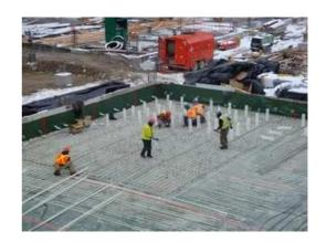
**Tension Lap Splice Length** Approximately 40 bar diameters for GFRP v.s. 30 bar diameters for steel .
